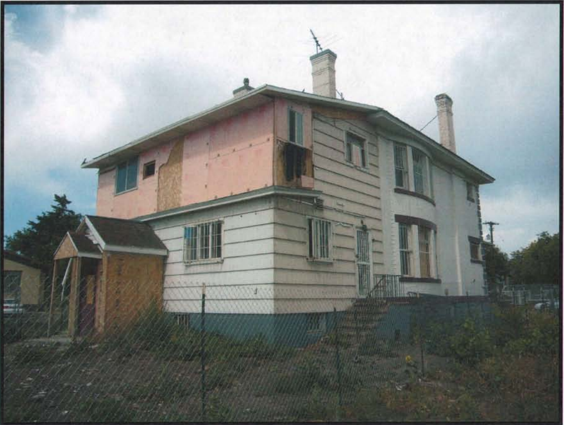
Rear and South Side of Taylor Residence
